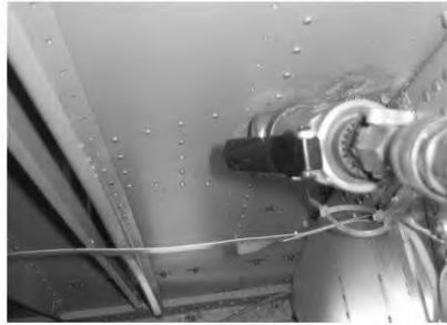
FIGURE 3 SUPPORT STRAP AND UPPER WING FORMER REMOVED
