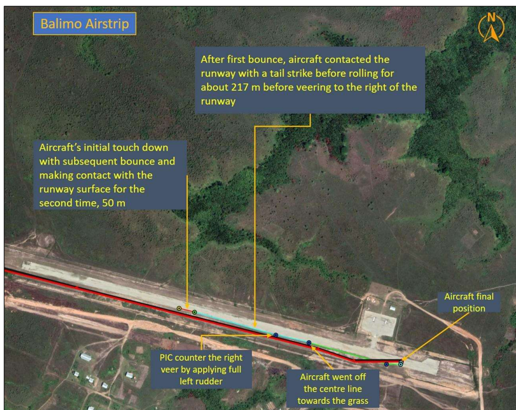
Figure 4. Assessment of Balimo Airstrip during the landing phase of the aircraft.
