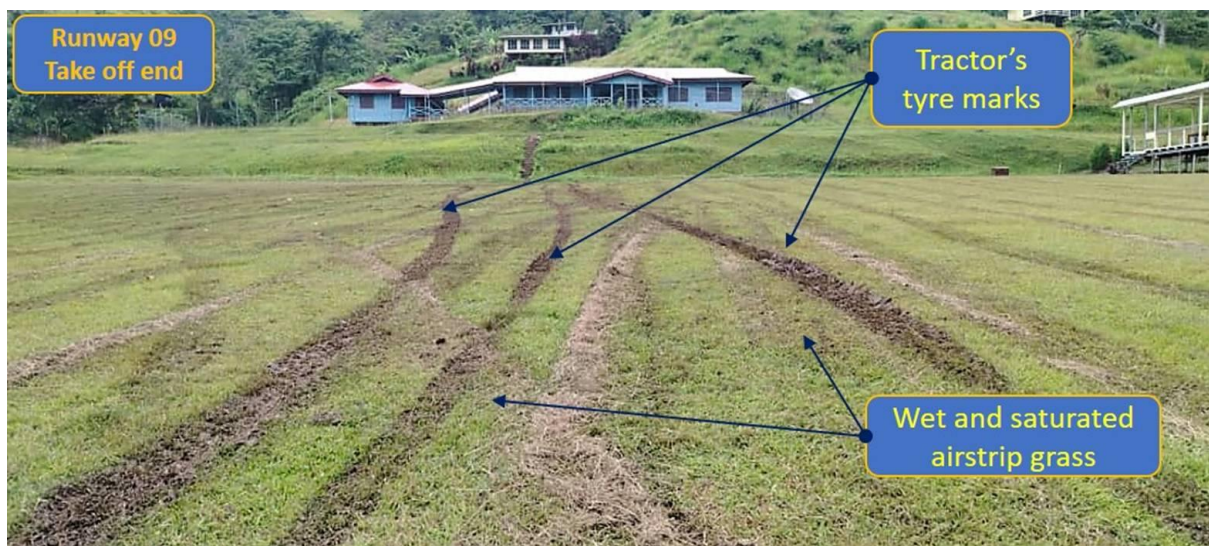
Figure 7. Strip surface conditions and tractor's tyre marks at Tapini Airstrip on the day of the accident.
